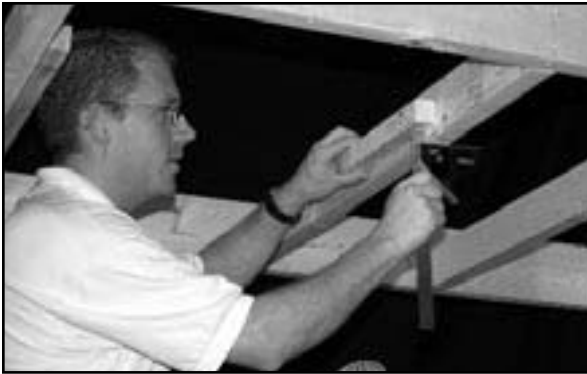
Figure 1: Installation of blocking for flush mounting of PIR to joists.
